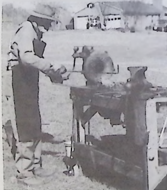
Jim McGavock forces air across the forge's coals which must reach 2,500 degrees in order to prepare iron for smiting.
